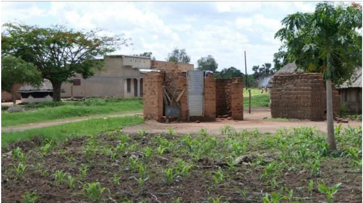
Photo Above: Latrine in Patongo TC with inadequate superstructure (no roof)
